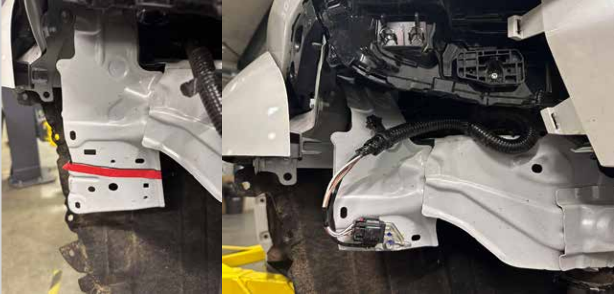
Figure 37: Left, mark and cut the structure. Right, reattach the electrical connector.
