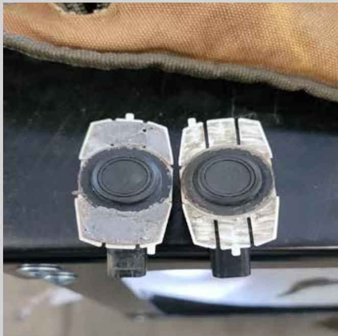
Figure 39: Label the location of each park sensor and remove the old double sided tape.
