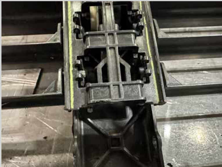
Figure 31: Bottom of the shutter mechanism trimmed flush.
