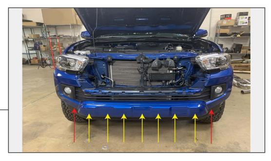
Remove (2) 8mm bolts, and (7) 10mm bolts from underneath the bumper.
