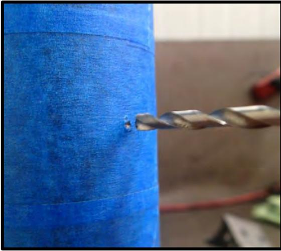
51. At the location of the center punch mark, use an Ø4mm (or similarly sized) drill bit to drill a pilot hole through the **REAR** face of the Bull Bar outer frame.
