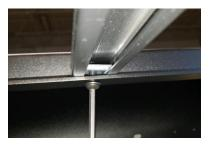
Add adhesive-back rubber isolators to cross bars, between plank mounting holes as shown below.
