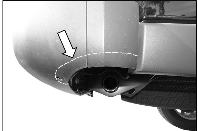
(Fig 10) Mark the cut line and cut the bottom edge of the factory bumper (Passenger/Right side shown)
