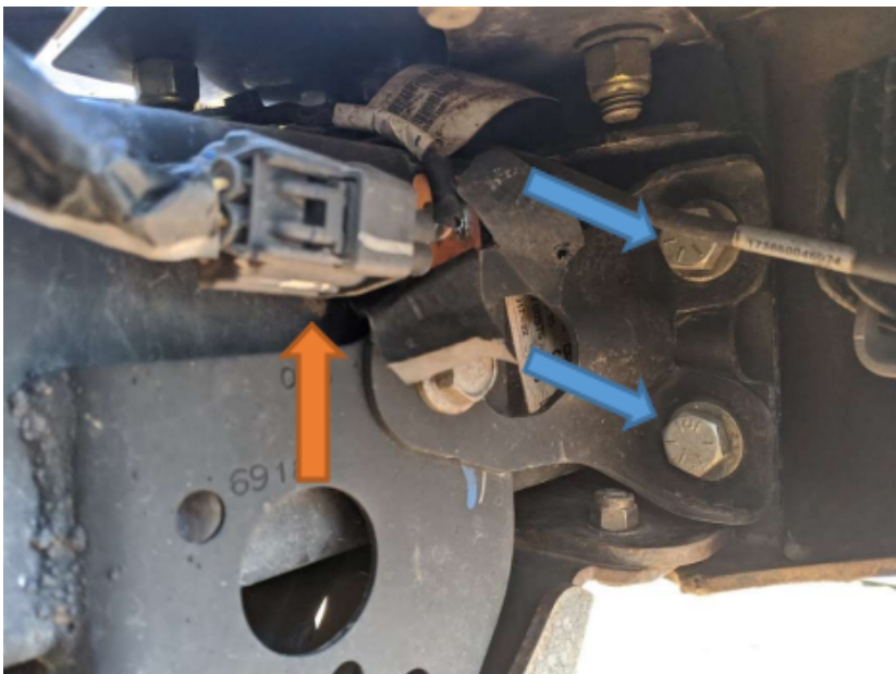
Figure 1: Passenger side frame rail at bumper mounting locations shown at blue arrows - There are 2 more on the other side of the frame rail not shown. Also shown (orange arrow) is the fog light connection that should be unplugged for this step.
