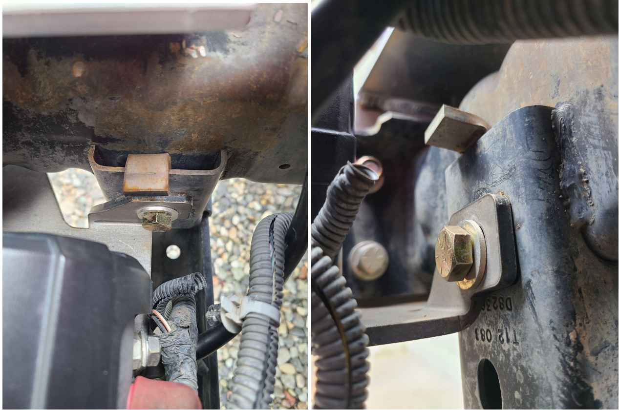
Figure 5: Nut stick “NV-JK-12 E” installed in passenger side frame through winch tray
