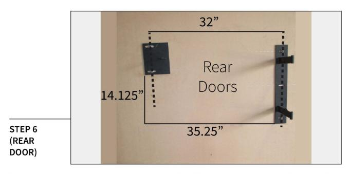
Locate a suitable location to mount the door brackets. The door brackets require (2) wall studs to secure the door, one for the hinge bracket and one for the latch bracket.
