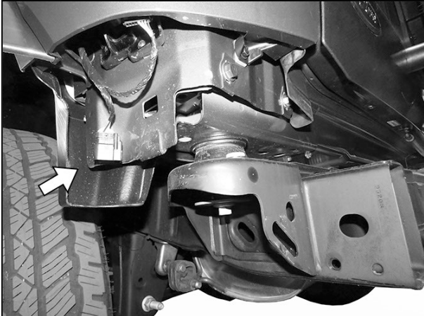
(Fig 1) Unplug all wiring harnesses leading to the rear bumper, (arrow-driver/left side pictured after bumper removal )
